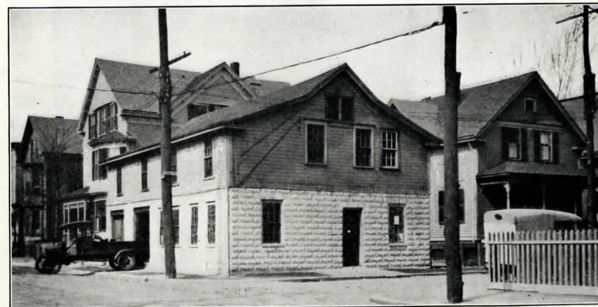
This Bottling Works is a Misplaced Use and Also Violates the Building Lines
